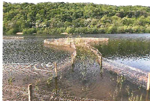
New reedbed at Bodenham
